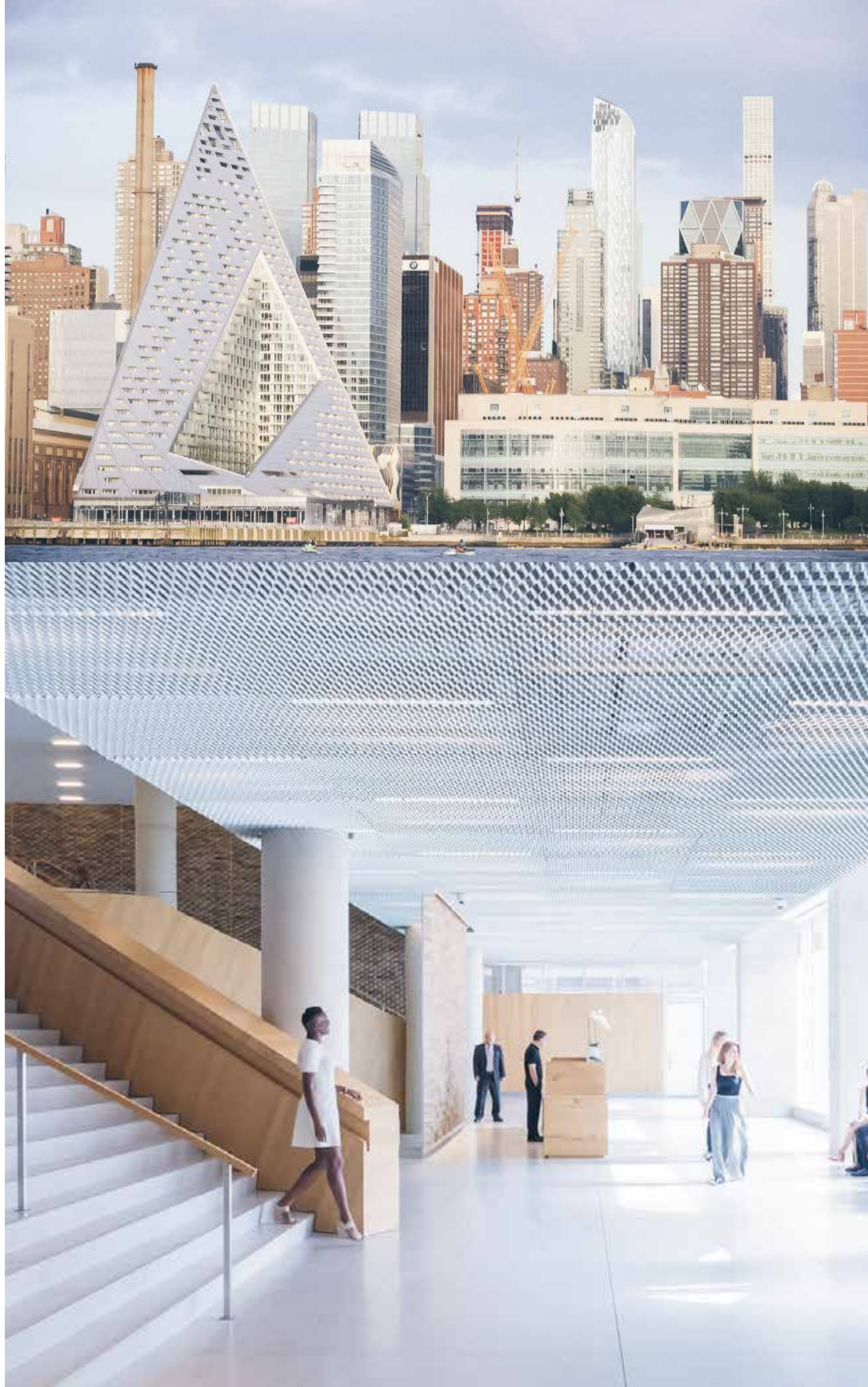
Via 57 West // New York, NY densified with LS // protected with Concrete Protector
