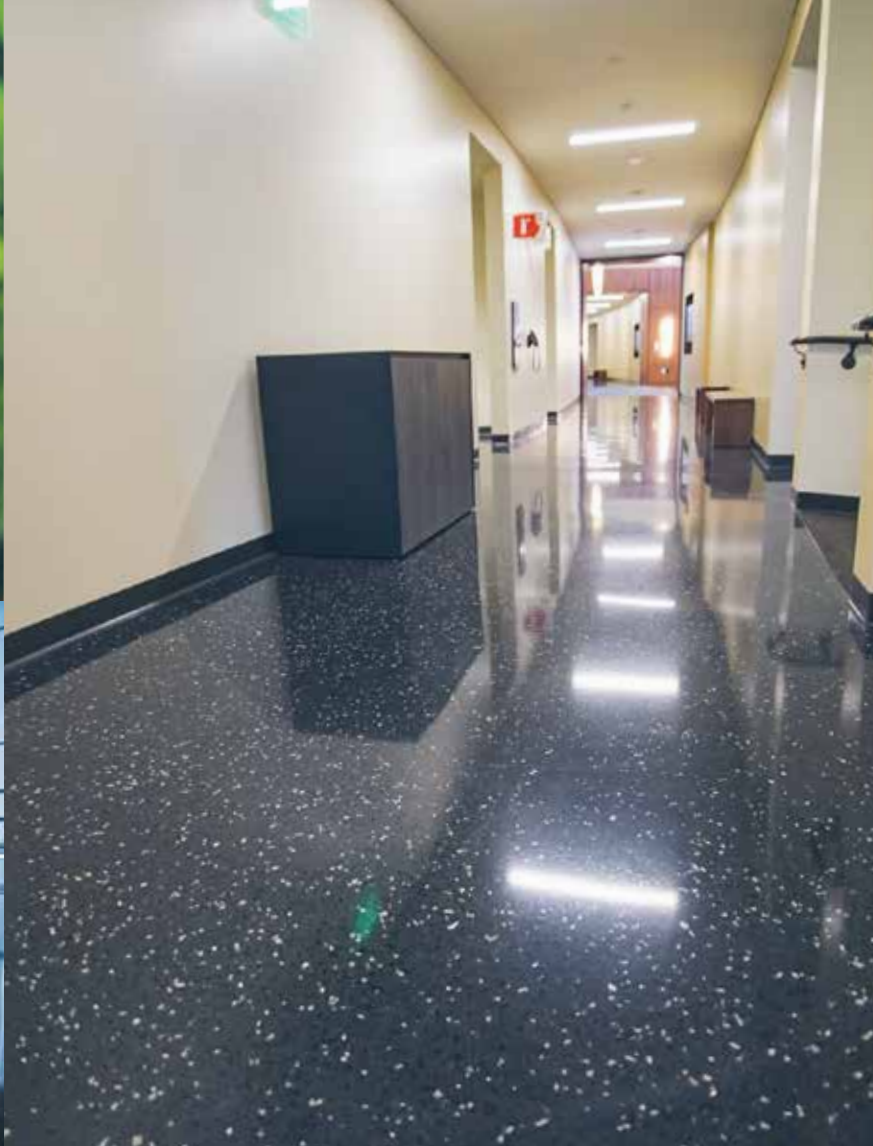
Skyline College Environmental Science Building // San Bruno, CA colored with Integral Color for Overlays in Black // densified with LS // protected with LSGuard
